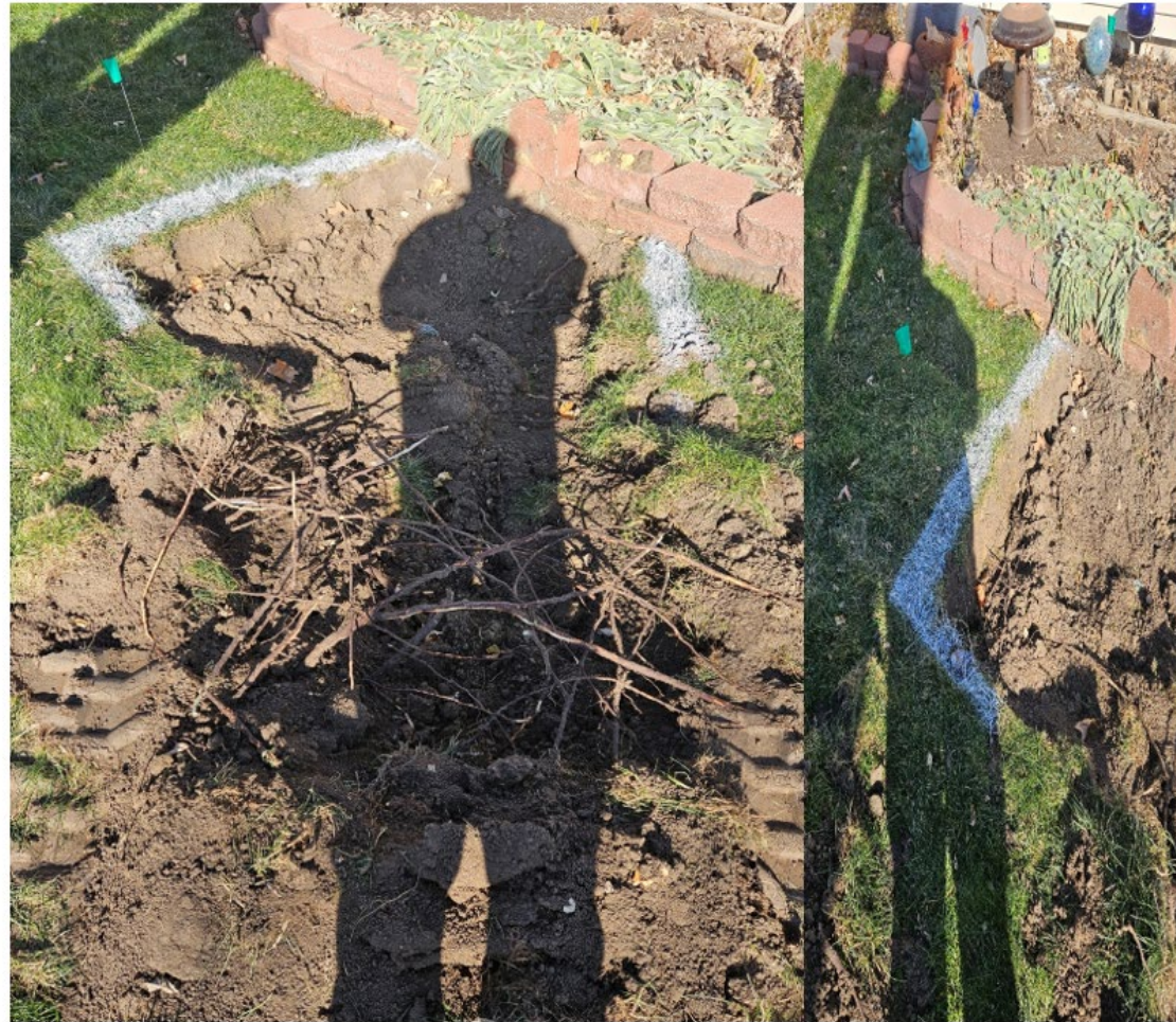
Images of the Excavation and hole in the ground.
